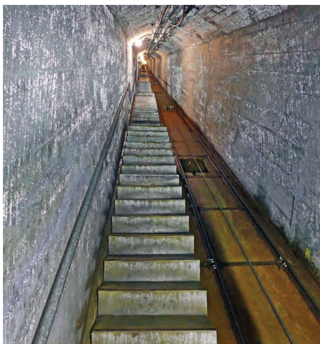
Fort Sasso da Pigna: The slope shaft linking the access tunnel with the higher gun casemate level
